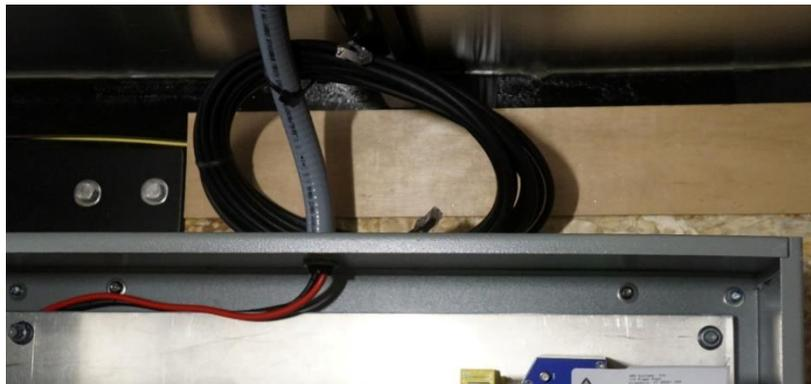
*When the trailer arrives from NRG, the 25' Ethernet cable can be found coiled and attached to the battery lead jacket on top of the electrical cabinet.*
