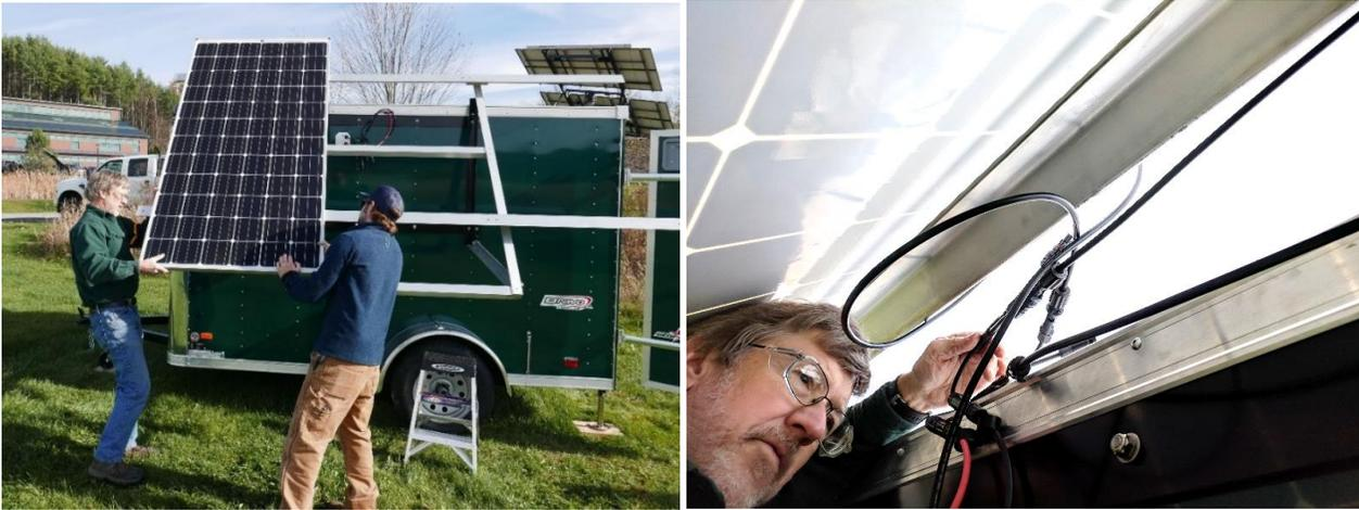
7. Connect each PV panel's male and female connectors to the trailer's male and female connectors.
