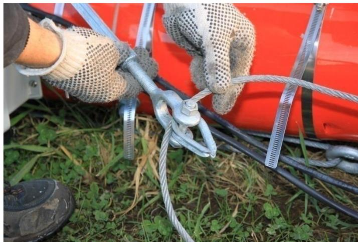
**Picture 3-52: Attach jumper strut cable to turnbuckle**
