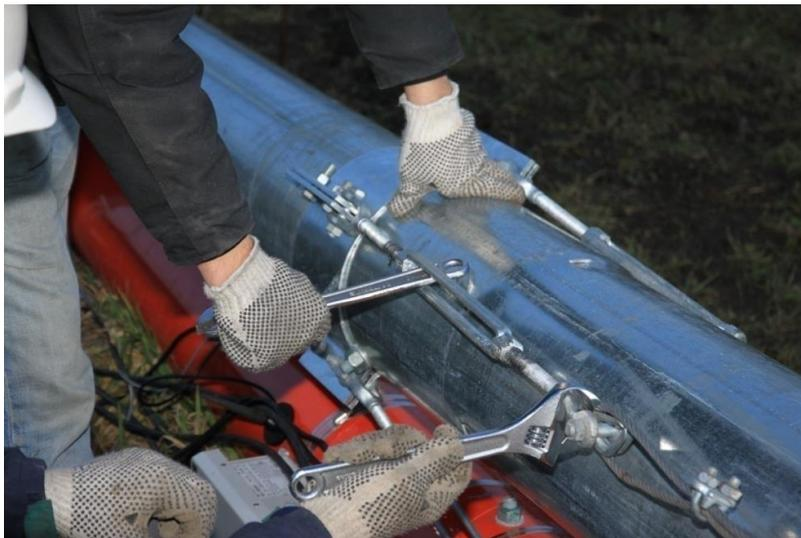
**Picture 3-79: Tightening turnbuckles**
