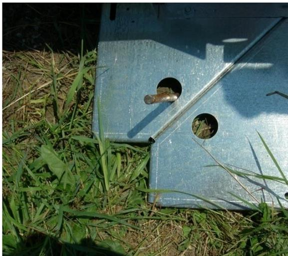
Picture 3-12: Ground Rod Placement
