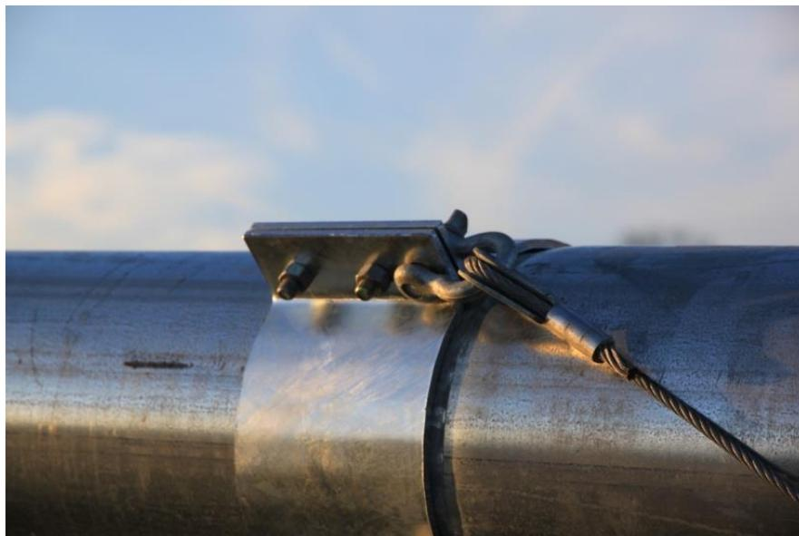
**Picture 3-48: Jumper strut cable attachment detail**
