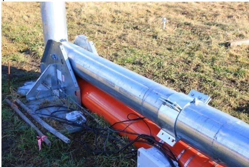
**Picture 3-40: Ginpole jumper strut end-flanges**
