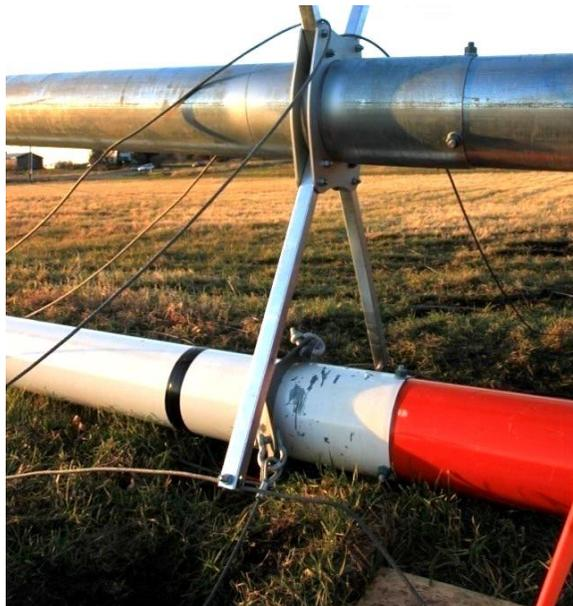
**Picture 3-49: Threading the jumper strut cable**
