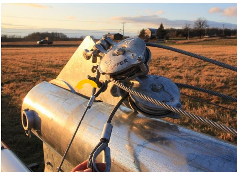
**Picture 3-75: Reeving through pulley #4**
