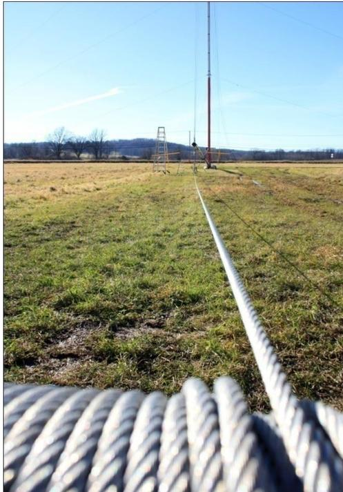
**Picture 3-68: Correct winch cable fleet angle**
