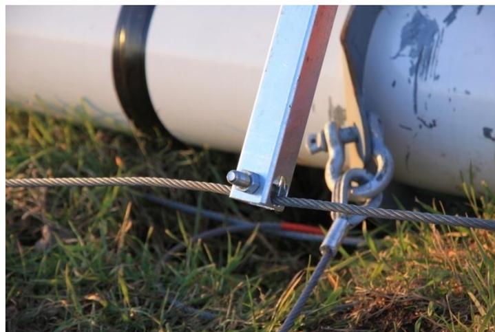
**Picture 3-50: Threading the jumper strut cable**
