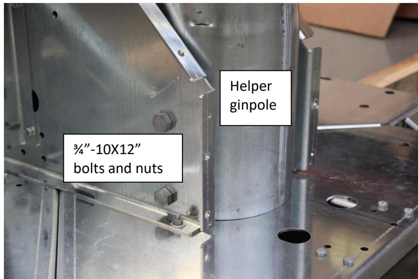
**Picture 3-62: Helper ginpole attached with bolts/nuts**
