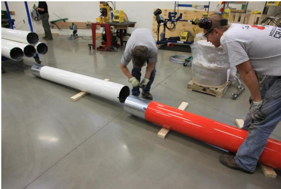
**Picture 3-16: Attach tower bolt/nuts**
