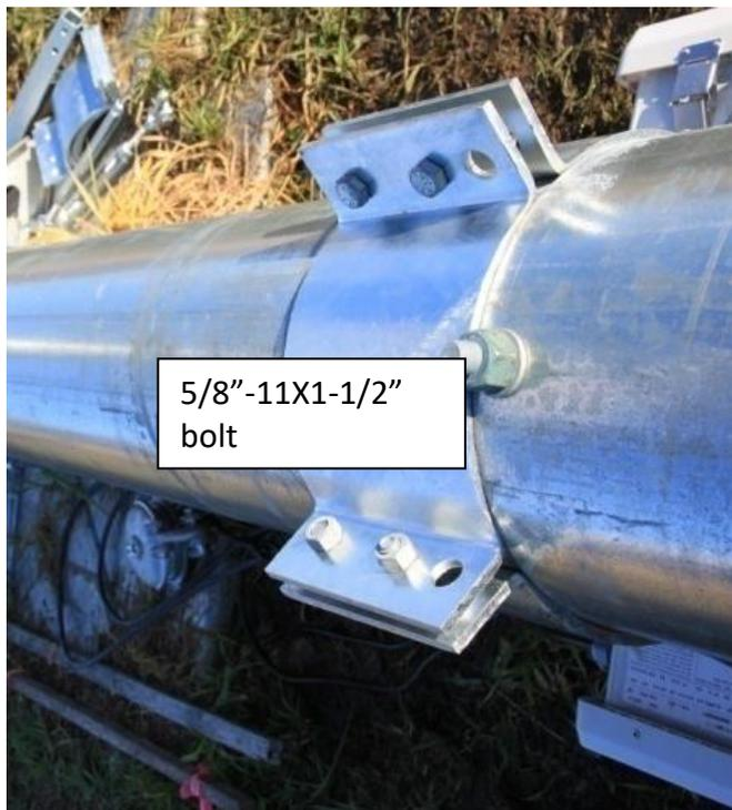
**Picture 3-41: Ginpole jumper strut end-flange bolts**
