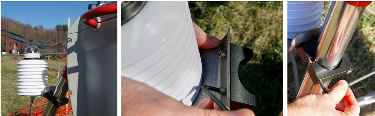
Figure 39: Installation of Met Sensor
