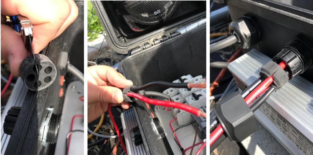
Figure 42: Cut gasket, place wires in gasket, secure with nut
