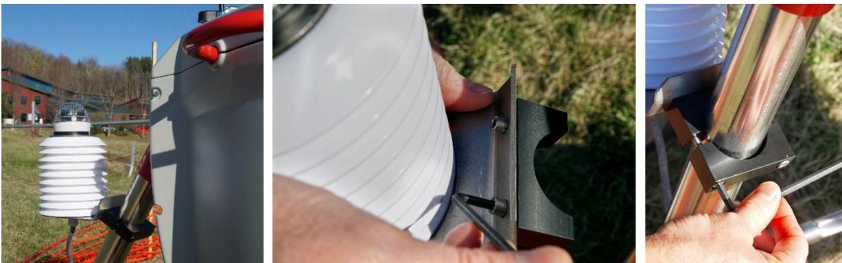
Figure 39: Installation of Met Sensor
