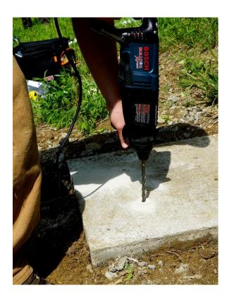
**Note**: The minimum embedment depth for 1/2" wedge anchors is 2.25 inches, but they **must** be installed deep enough to ensure that only the threaded portion of the anchor is exposed (typically 3" deep).
