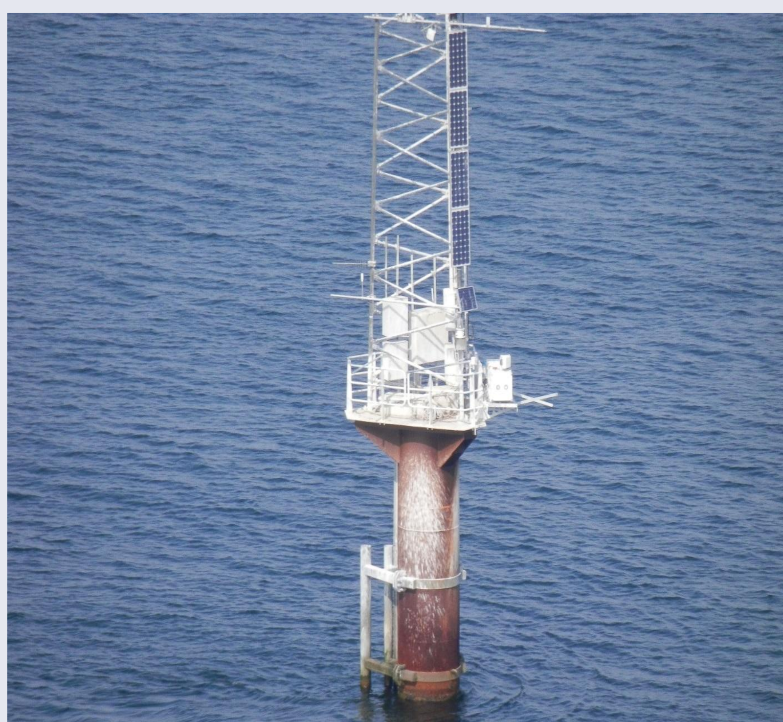
Windcube located on Met Mast platform
