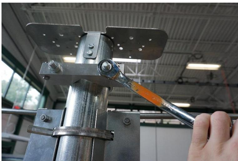
Figure 1-3: Mounting the upper U-bolt
