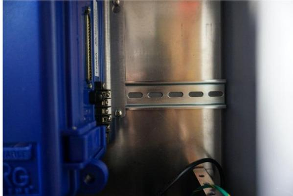
Figure 2-2: DIN rail mounted to shelter box backing plate.
