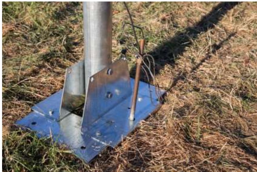
Figure 2-14: Installed ground rod
