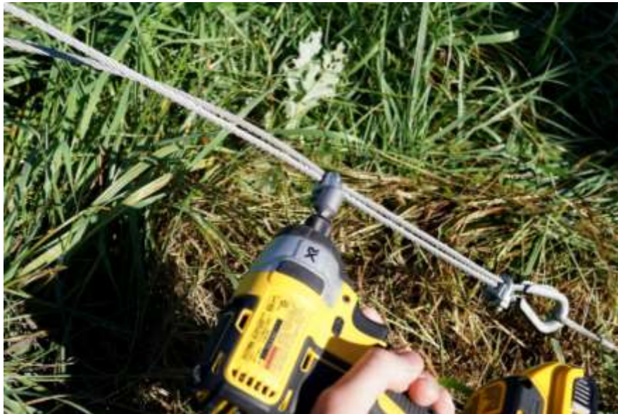
Figure 2-12: Guy wire secured by wire rope clips. Duckbill anchor wires have a thimble preinstalled.
