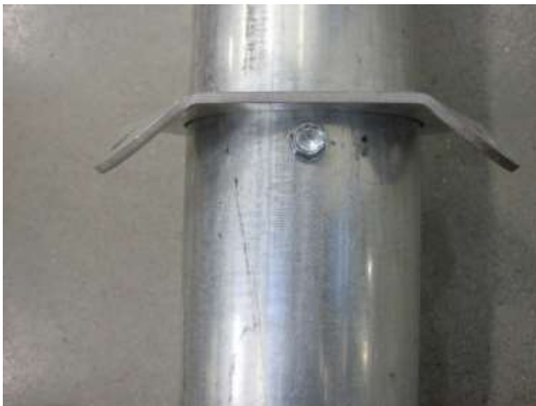
Figure 2-4: Guy ring installed onto tower tube to the preinstalled screws
