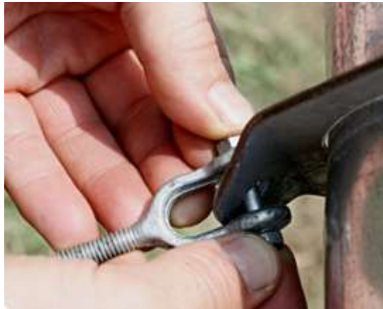
Figures 2-10 & 2-11: Turnbuckle attachment points to guy ring and guy wires
