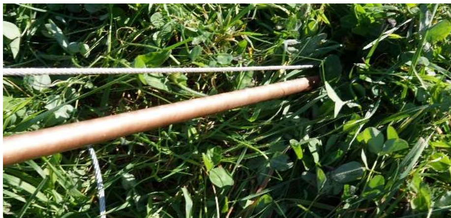
Figure 2-8: Pound Duckbill anchors into place using the ground rod
