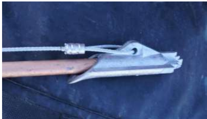
Figure 2-7: Placing the Duckbill anchor onto the tip of the ground rod
