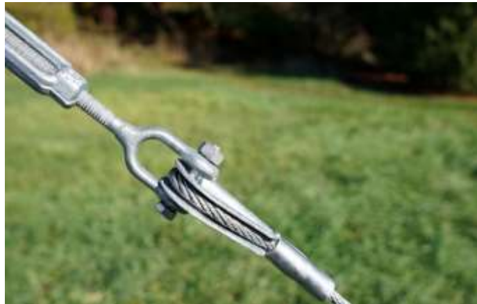
Figures 2-10 & 2-11: Turnbuckle attachment points to guy ring and guy wires
