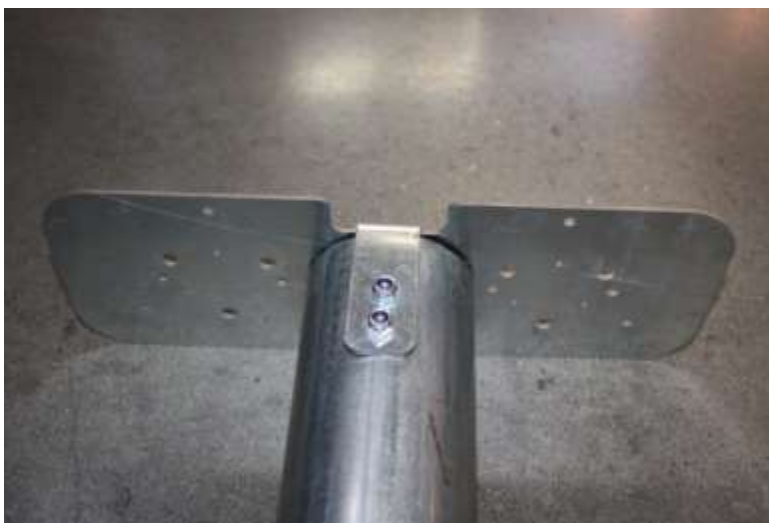
Figure 2-5: Top plate installed
