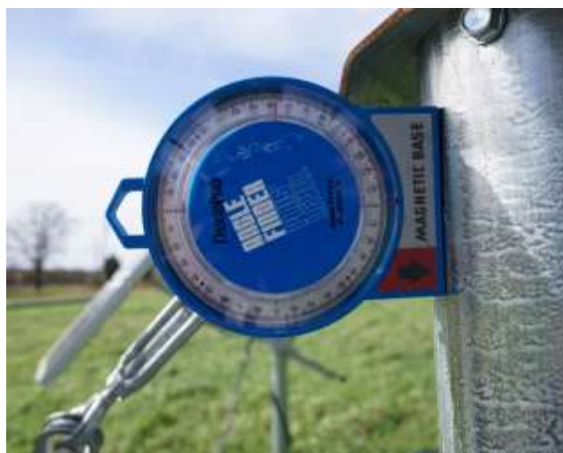
Figure 2-13: Plumb the tower with the angle meter
