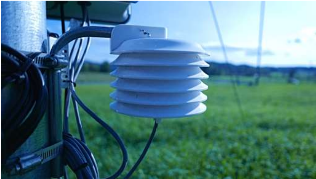
Figure 2-20: NRG 110S Temperature sensor attached to the tubular tower with band clamps.
