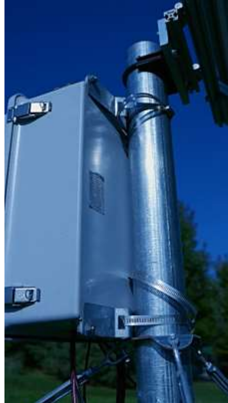
Figures 2-18 & 2-19: Shelter box brackets and attachment to the tubular tower.
