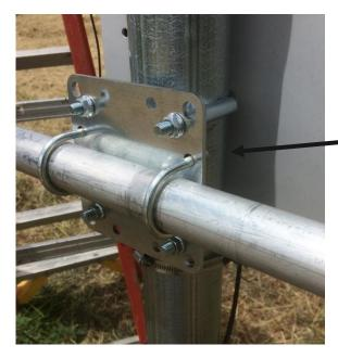
Attach upper PV boom 1.27m (50 inches) up the tower on the south side
