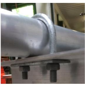
Using a ½ inch open ended wrench, tighten down all U-bolts when desired PV angle is obtained.
