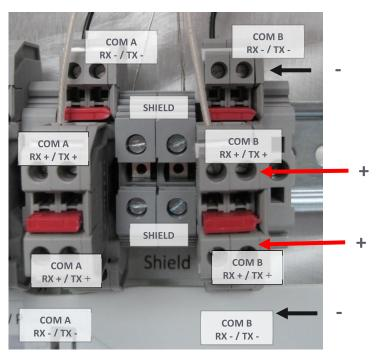
Note: with this DIN Rail Mounted Terminal Style, "front" terminals are "+" and "back" terminals are "- ".
