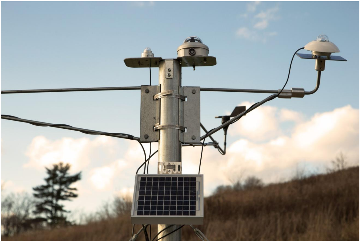
Figure 2-15: Secure Booms to Tower
