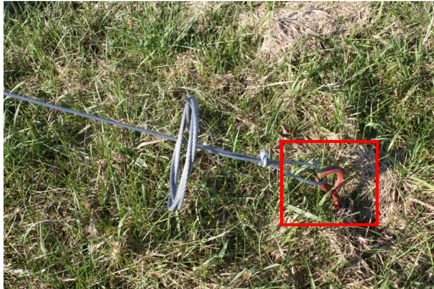
Figure 2-3: Anchor Installation
