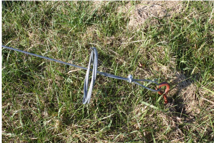
Figure 2-11: Attach Guy Wire to Anchor
