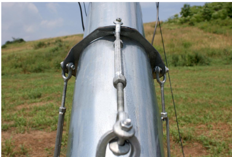
Figure 2-10: Attach Turnbuckle to Guy Wire's Thimble
