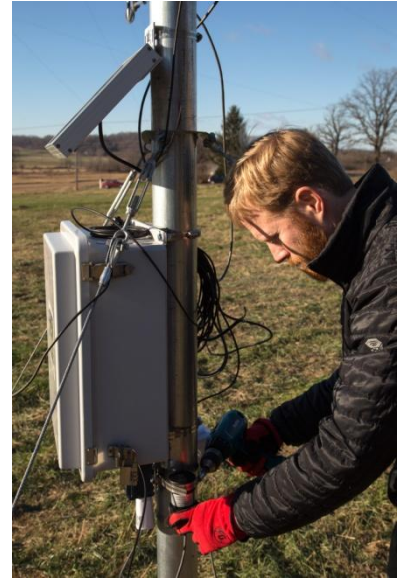
Figure 2-19: Tighten sensors
