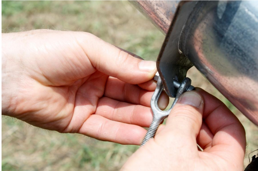
Figure 2-9: Attach Turnbuckle to Guy Ring
