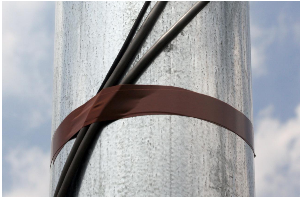
Figure 2-20: Wrap Sensor Cables around Tower
