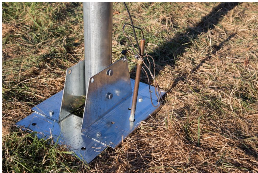
Figure 2-8: Drive Ground Rod
