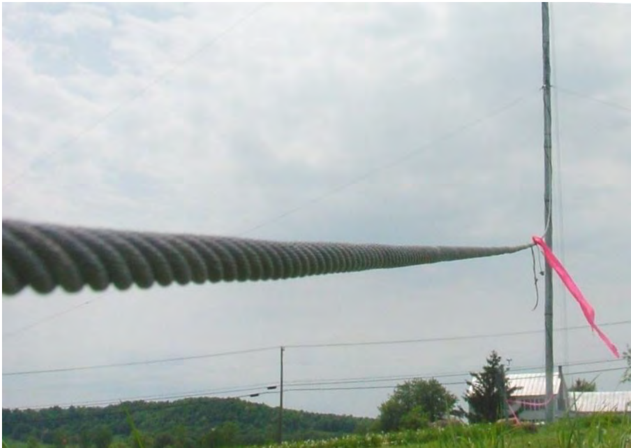
Picture 95: Level 1, Guy Sag = 2.5 Tubes
