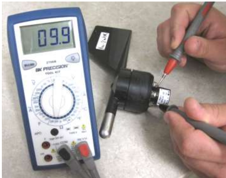
Test 1: Measure across (+) and (-)
