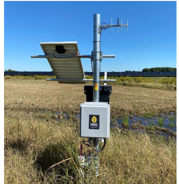
Flood detection system at Hillcrest Solar Project, Ohio.
