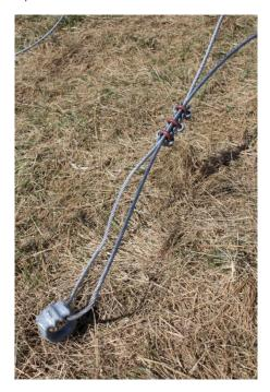
3) Tension the cables using the come-along and the Chicago grips provided with the 80m tower by securing the Chicago grip onto the cable about 3.5 feet from the anchor eye. Secure the slack end of the comealong to the shackle on the shaft of the anchor, and secure the other end to the Chicago Grip.
