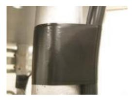
3) Wrap three full turns of one inch Scotchwrap<sup>™</sup> Filament #890 tape (or equivalent) over the Scotchwrap<sup>™</sup> #50 tape.
