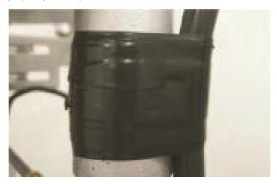
5) Avoid contact with the guy rings by enforcing slack in the cable over the guy rings. This will avoid damage to the cable by preventing contact with the guy rings.
