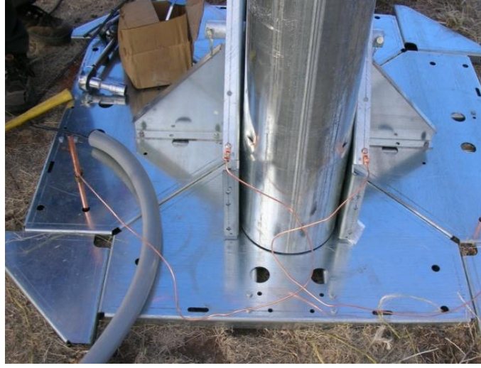
Picture 3-13: Tower Grounding
