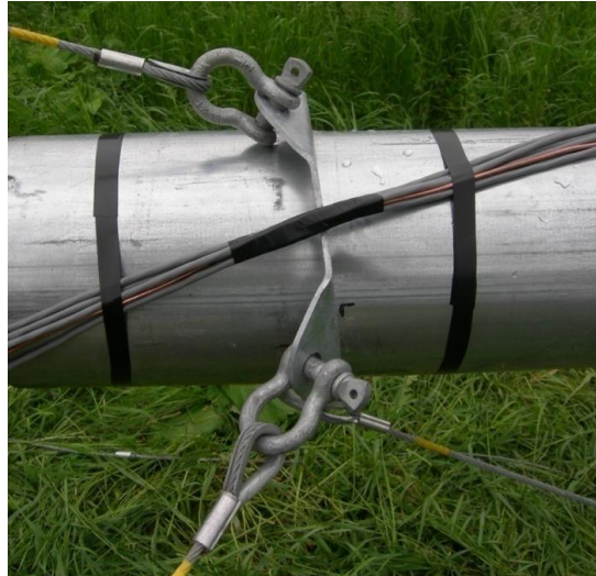
Picture 3-29: Cable protection
