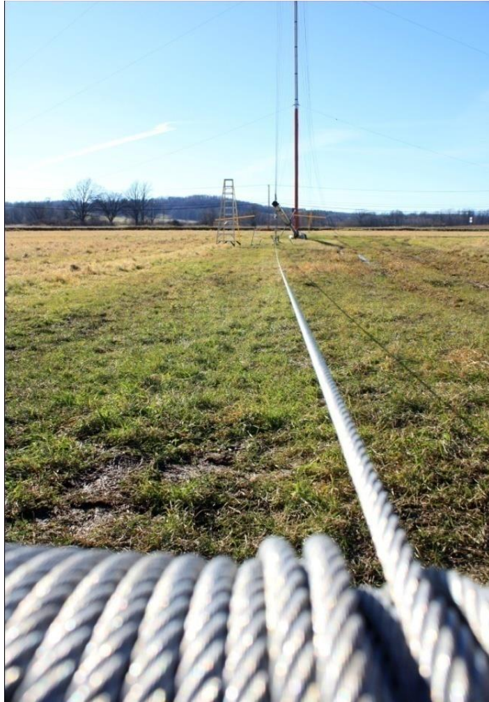
Picture 3-69: Correct winch cable fleet angle
