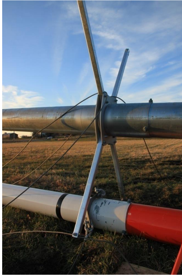
Picture 3-50: Threading the jumper strut cable
