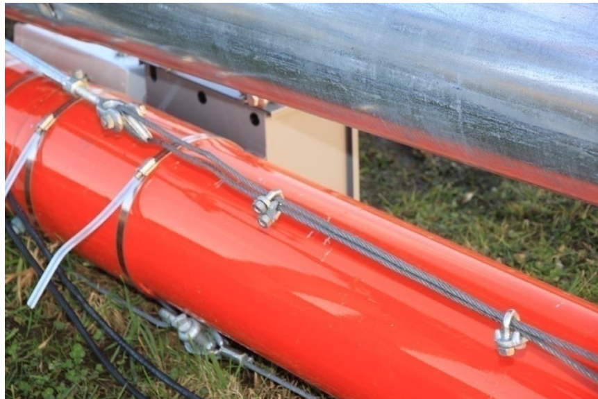
Picture 3-52: Attach jumper strut cable to turnbuckle
