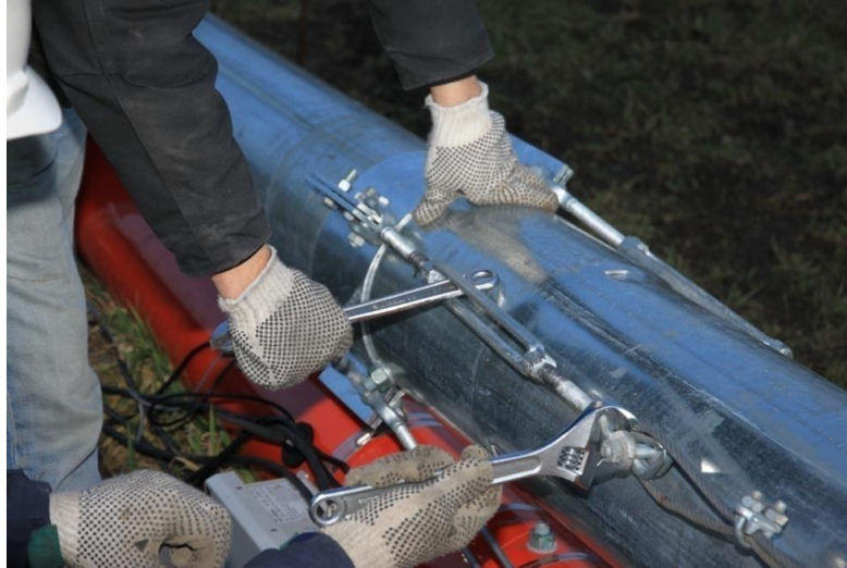
Picture 3-80: Tightening turnbuckles
