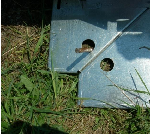
Picture 3-12: Ground Rod Placement
