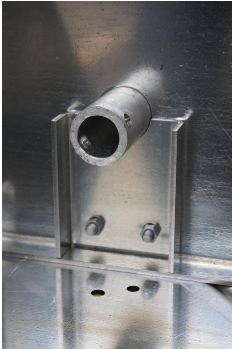
Picture 3-10: Baseplate Assembly
