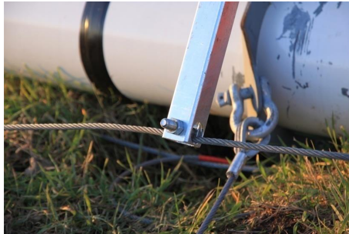
Picture 3-51: Threading the jumper strut cable
