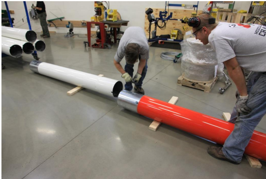
Picture 3-16: Attach tower bolt/nuts
