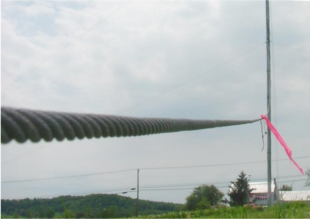
Picture 4-8: Level 1, guy sag = 2.5 tubes – TOO LOOSE!
