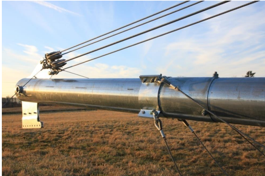
Picture 3-48: Jumper strut cable attachment
