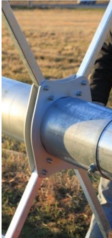
Picture 3-47: Jumper strut alignment
