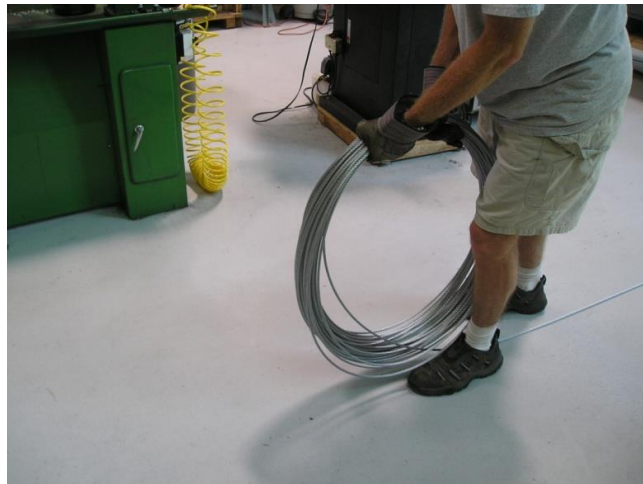
Picture 3-31: Unroll guy wires CORRECT
