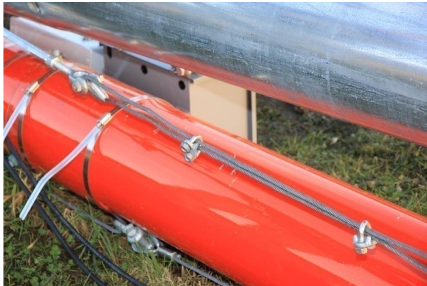
Picture 3-52: Attach jumper strut cable to turnbuckle
