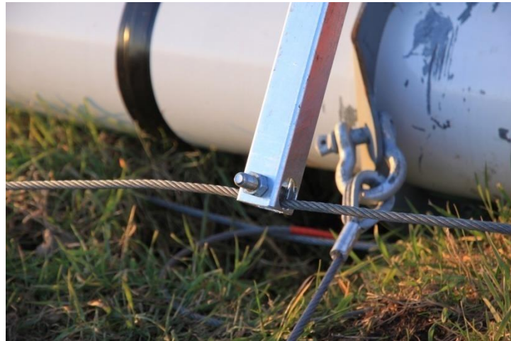
Picture 3-51: Threading the jumper strut cable
