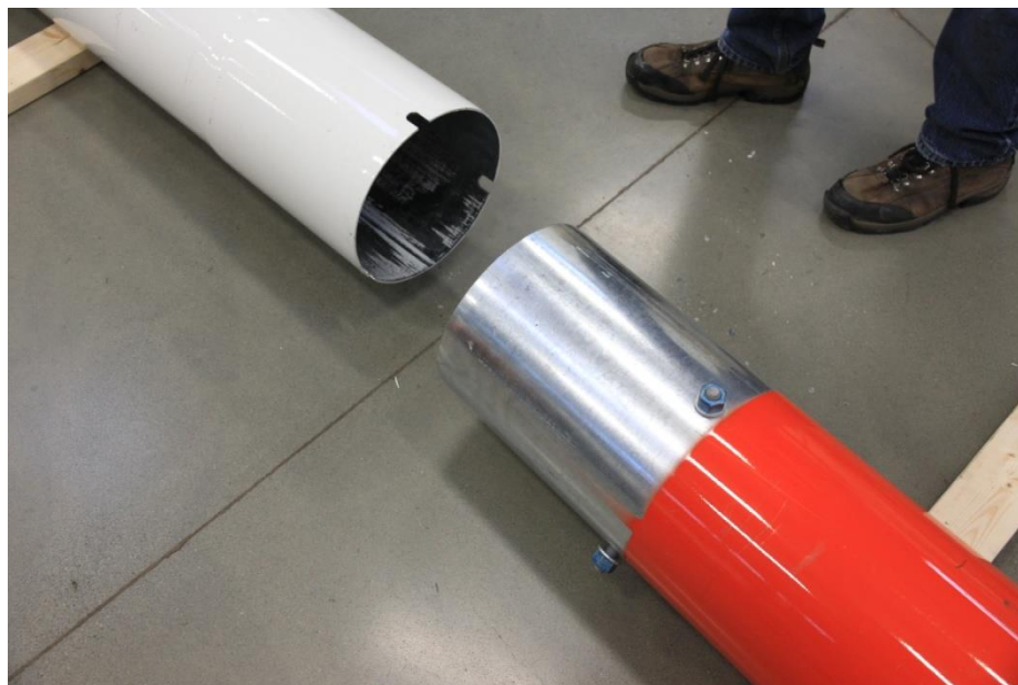
Picture 3-17: Tubes ready to be connected, weld seam down
