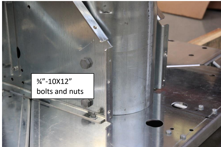
Picture 3-63: Helper ginpole attached with bolts/nuts
