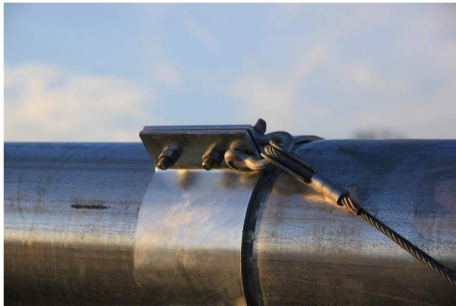
Picture 3-49: Jumper strut cable attachment
