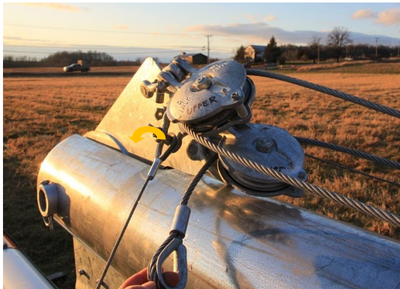
Picture 3-76: Reeving through pulley #4
