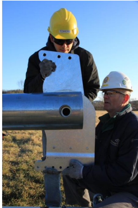
Picture 3-55: Ginpole rocker plate assembly
