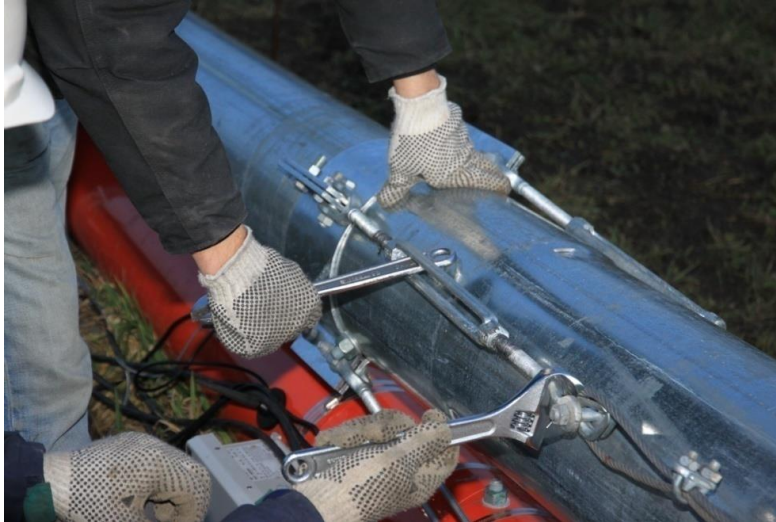
Picture 3-80: Tightening turnbuckles
