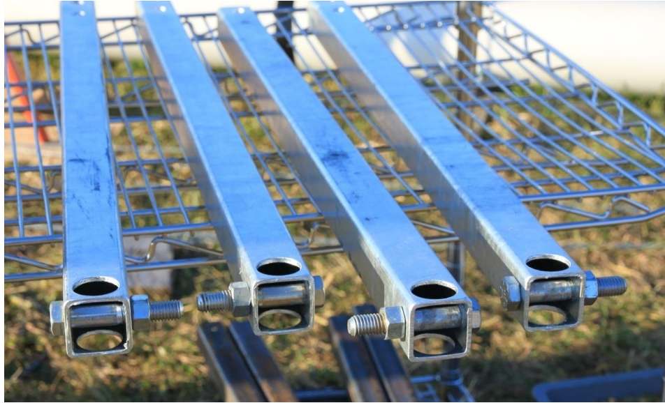
Picture 3-45: Install bolts/nuts onto jumper struts
