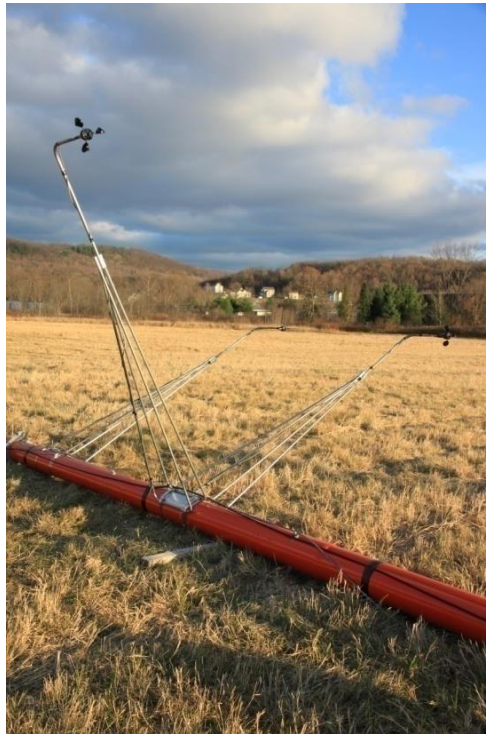
Picture 3-28: Boom installation
