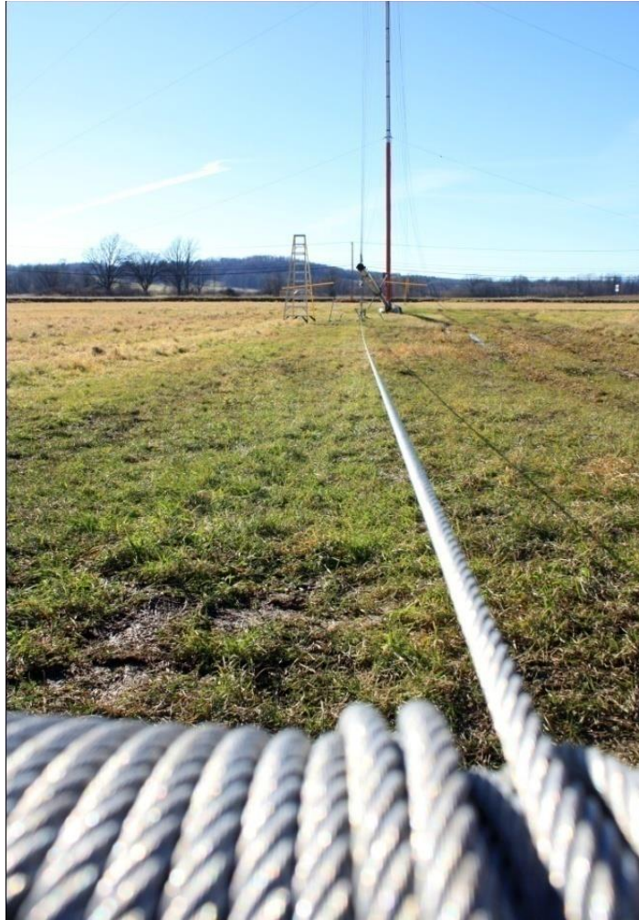
Picture 3-69: Correct winch cable fleet angle
