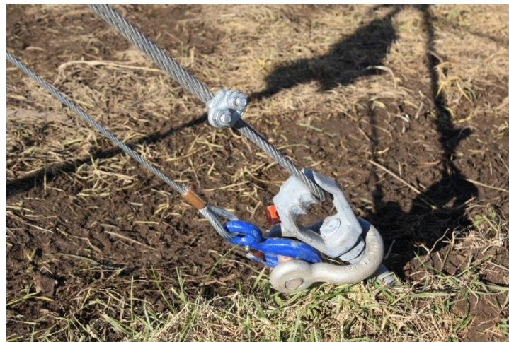
Picture 4-4: Use a shackle to aid in attaching come-along without pinching cables
