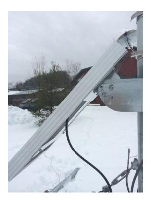
When installing the PV panel, select a location that will minimize shading. Even the shade from a cable can greatly reduce the output of a PV panel. Coil and secure extra cables with electrical tape to prevent them from flapping in the wind.
