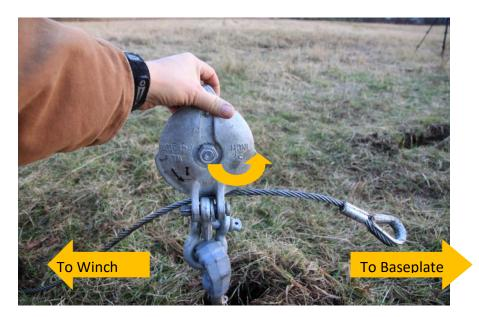
Picture 3-72: Reeving through pulley #1
