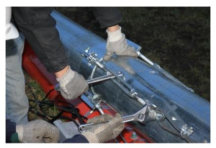
Picture 3-79: Tightening turnbuckles
