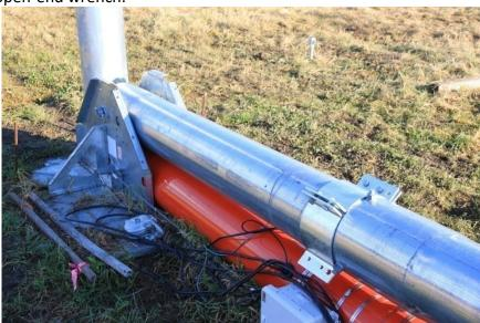
Picture 3-40: Ginpole jumper strut end-flanges
