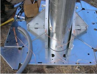
Picture 3-12: Ground Rod Placement
