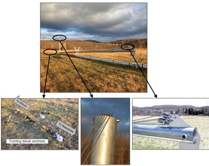
Picture 3-70: Correct reeving of the winch cable
