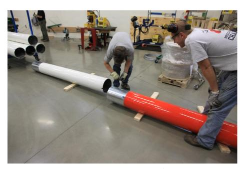
Picture 3-16: Attach tower bolt/nuts
