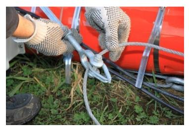
Picture 3-52: Attach jumper strut cable to turnbuckle
