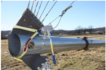
Picture 4-10: Set up for transfering lifters to their storage anchor
