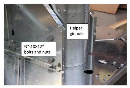
Picture 3-62: Helper ginpole attached with bolts/nuts
