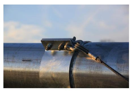
Picture 3-48: Jumper strut cable attachment detail
