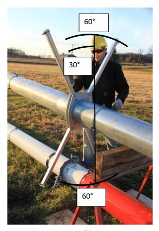
Picture 3-45: Install jumper struts
