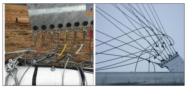
Picture 3-58: View of front guy wires attached to lifters (80 m tower) before and after tower raising
