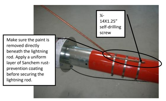
Picture 3-27: Proper lightning spike installation
