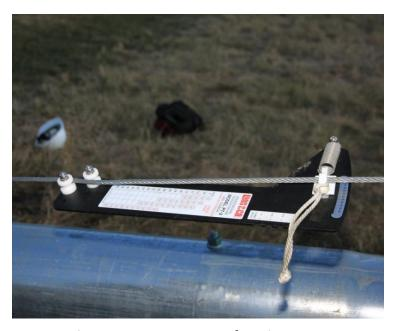
Picture 3-80: Correct use of tension gauge
