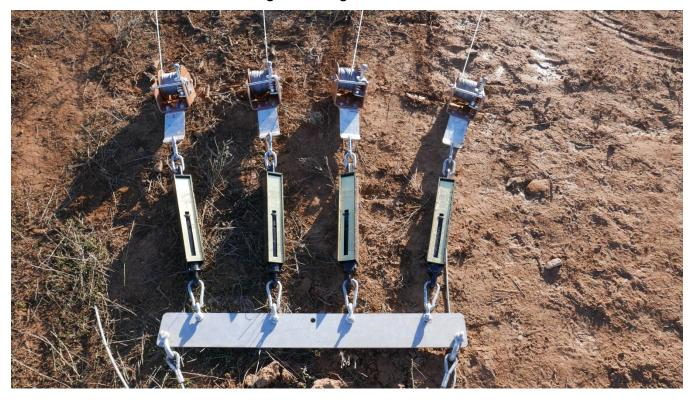
Picture E-9: Set-up of Back Guywire Tensioner (Picture shows 80m tower set-up using 4 worm gears on each side. Super 60 utilizes 3 worm gears on each side).
