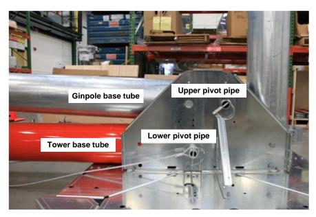
Picture 3-63: Complete baseplate and tower assembly ready for raising
