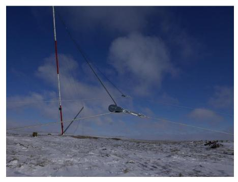
Picture E-4: Leader cables attached to back guywires using pulleys
