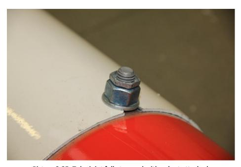
Picture 3-25: Tube joint fully torqued with palnut attached
