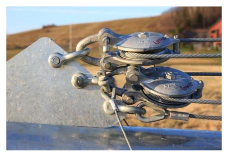
Picture 3-59: Correct block pulley assembly
