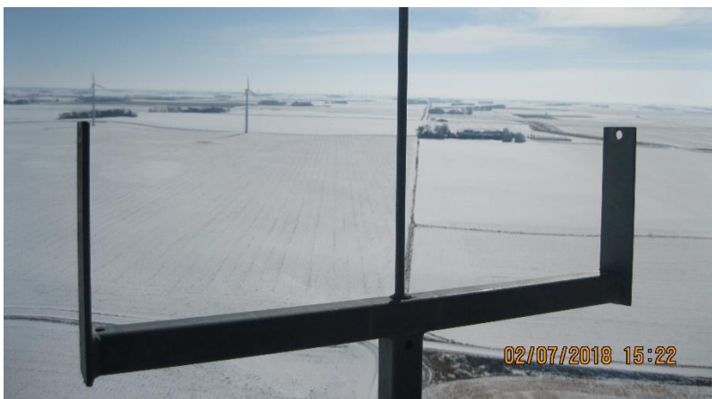
Figure 2 | Met mast after removing old sensors
