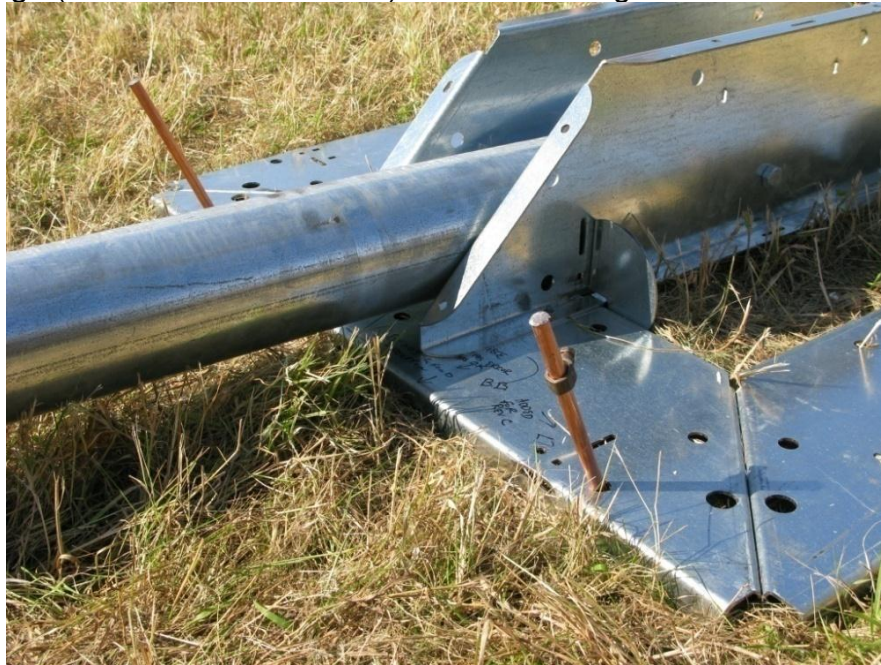
Figure 7 Install the Base Tube
