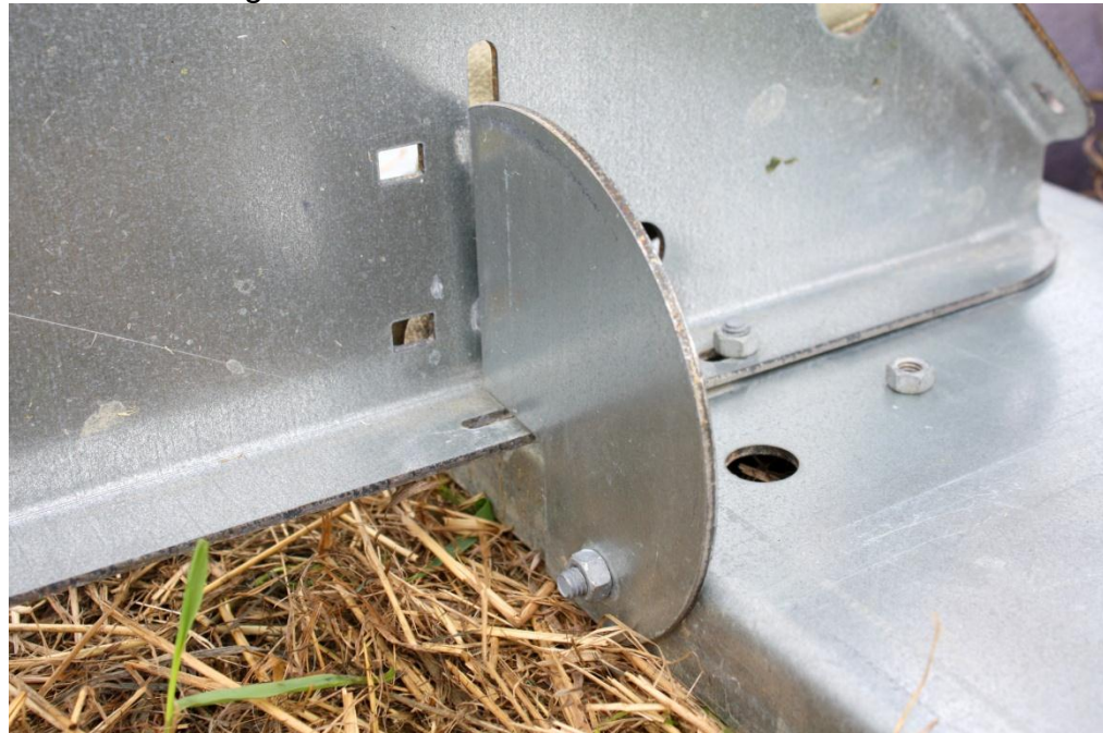
Figure 5: Secure Gusset to Horizontal Baseplate
