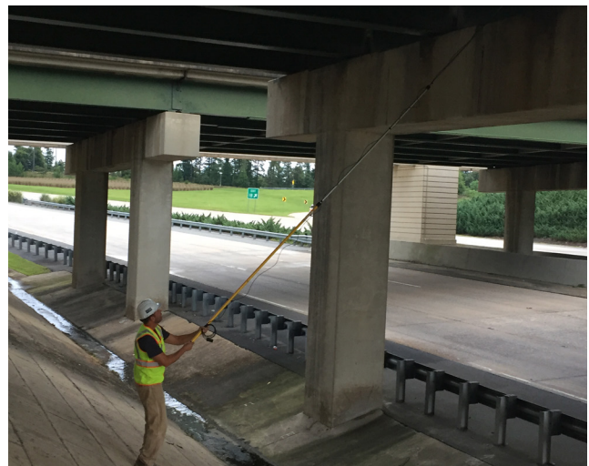
Figure 8. Borescope Inspection of Expansion Joint
