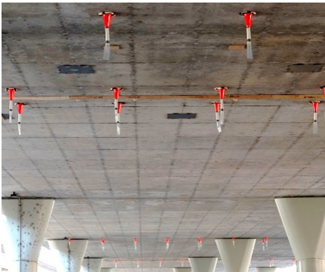
Figure 3. Physical Exclusion Methods Used by California Department of Transportation, Sacramento, CA.
