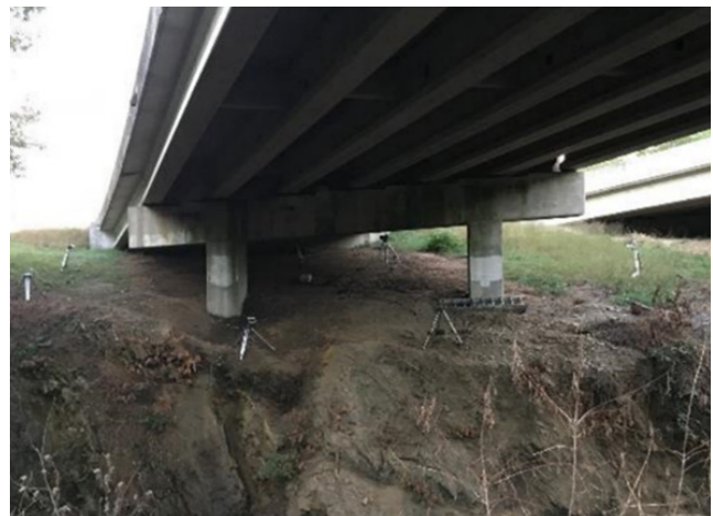
Figure 10. BDU Arrangement Around Expansion Joint
