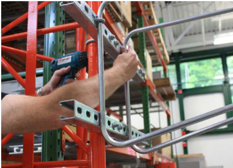
Figure 7 | Attaching the boom to the brackets using U-bolts
