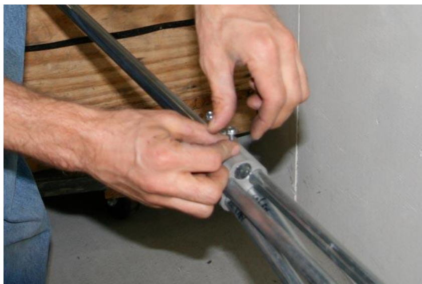
Figure 2 | Installing the self-tapping screws
